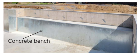
Possibility of integrating a concrete bench
