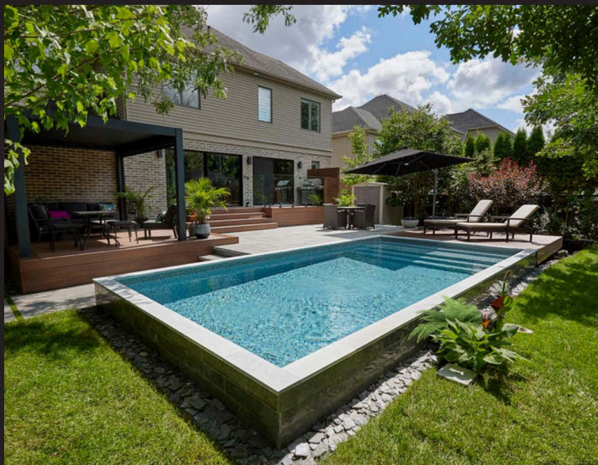
21 TRÉVI EUROPEA Built-in pool / Reinforced concrete
